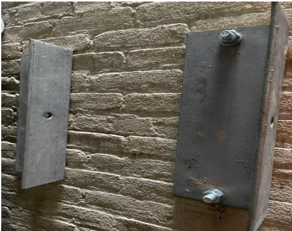
Anchor plates installed awaiting pull test Thursday 3/30/23
