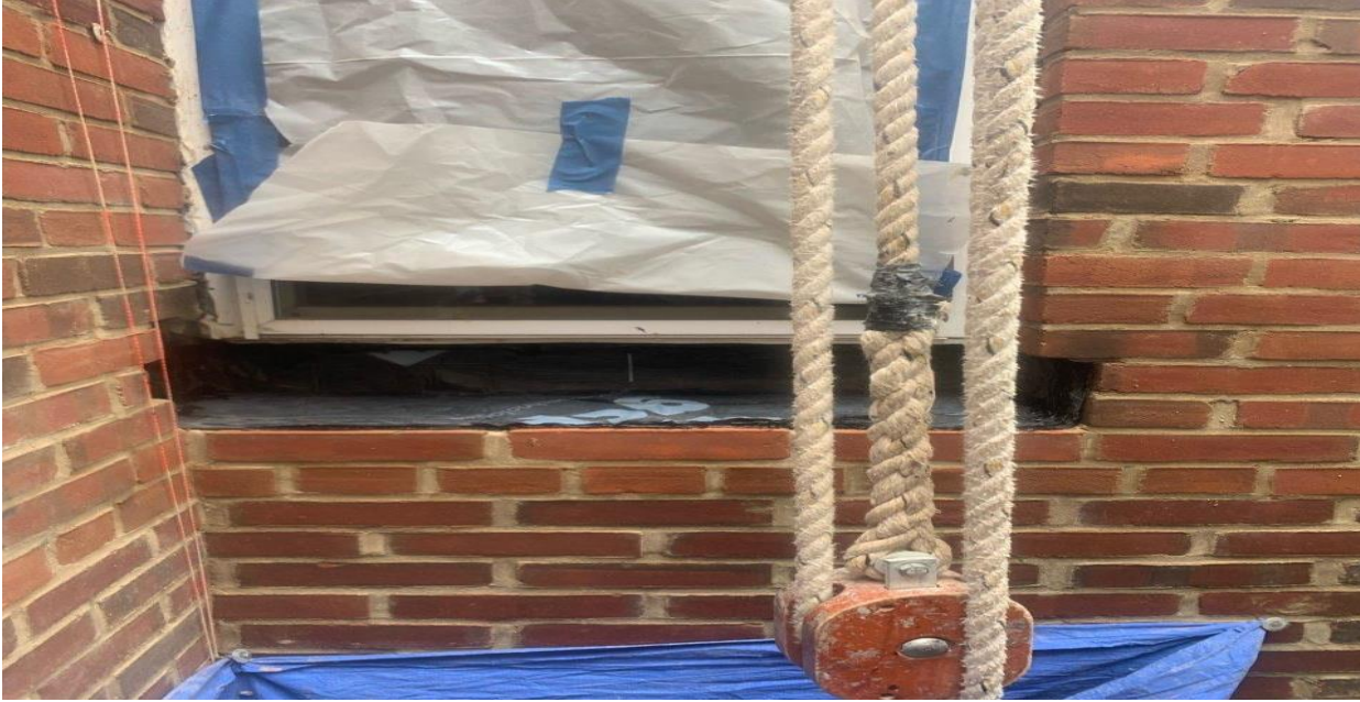
Sill waterproofing installed
