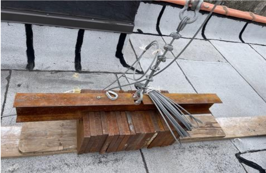
Anchor plates installed awaiting pull test Thursday 3/30/23
