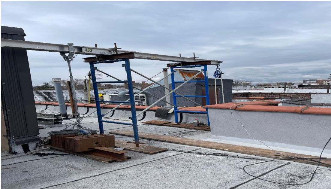
Material Hoist installed
