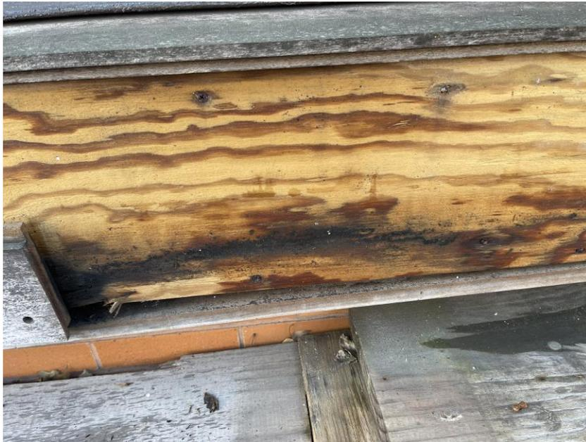
**Existing conditions of plywood that is being removed. Large gaps, mold, and no waterproofing installed.**
