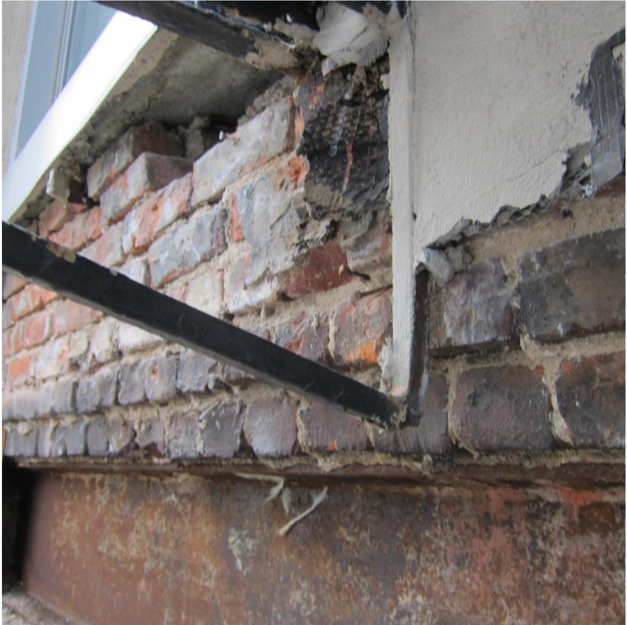
Photo 3: Close view of the probe opening on the 8 th Floor.
