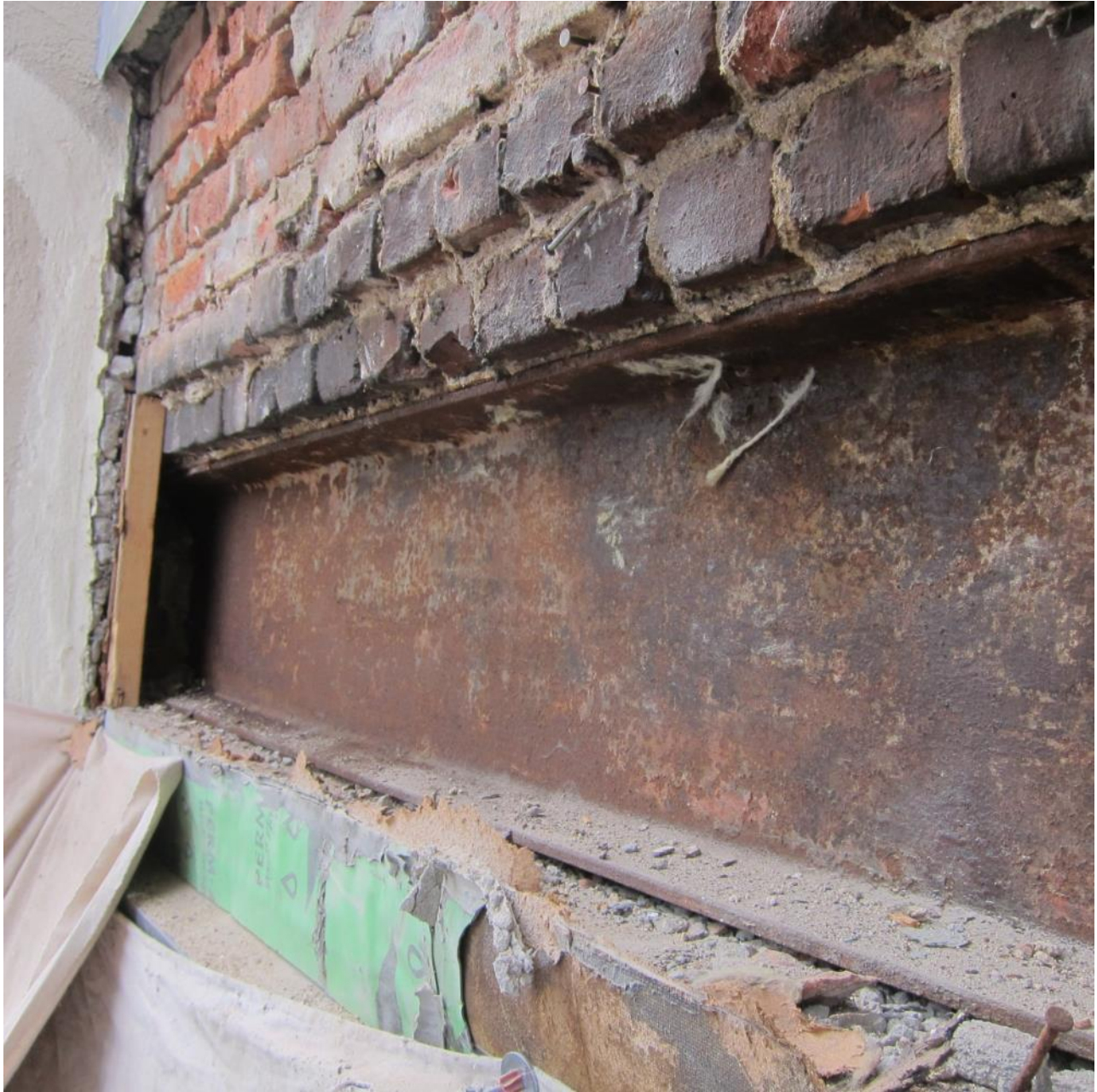
Photo 2: Close view of the probe opening on the 8 th Floor.
